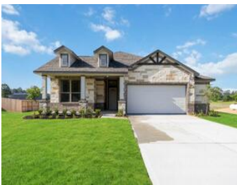
301 Barton Place Drive Cleveland, Texas 77327
