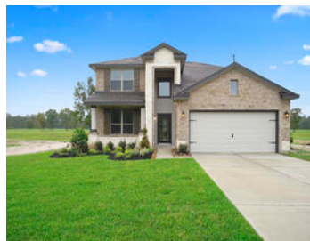
201 Barton Place Drive Cleveland, Texas 77327
